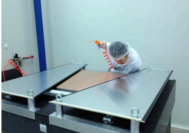
Figure 83: Epoxying the anode wires on the wire mounts with protecting covers in place.
